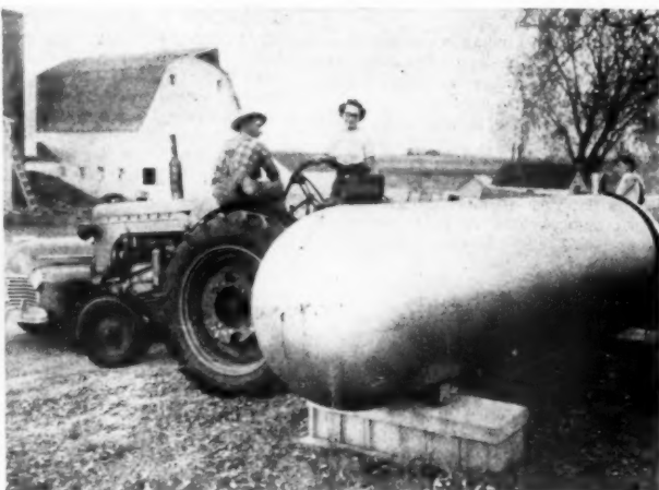
DOMESTIC USE. —A farmer is shown fueling his L.P.G.-powered tractor from the same tank that supplies L.P.G. for heating and cooking purposes in his home. Other farm uses include pumping and irrigation, brooder heating, and flame weeding.
